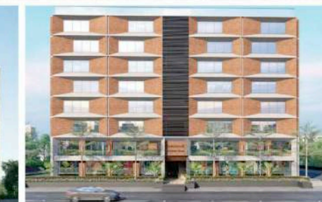
Indraprasth Business House (Showrooms & Offices)
